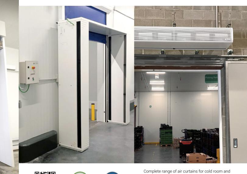
TRIOJET air curtain system is specially designed for freezers with large temperature differences. Ice, snow and fog are reduced, decreasing the risk of accidents while increasing energy savings and correct preservation of frozen products.
